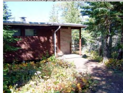
Housekeeping Cabin at Rock Harbor
