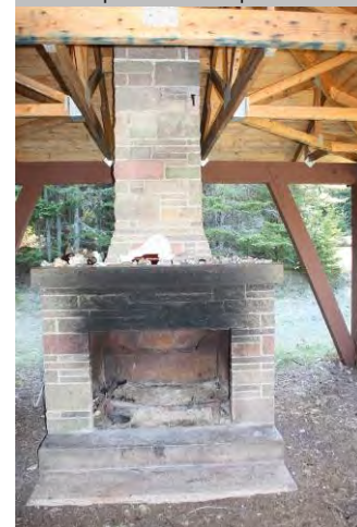
Fireplace under the pavilion.
